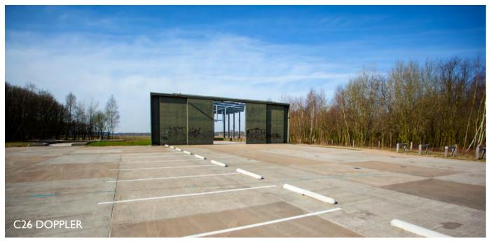
In this monumental building, a so called 'run-up', jet engines of among others the F-16 fighter jets were tested. Because of the heavily insulated cladding, the building was virtually soundproof.
