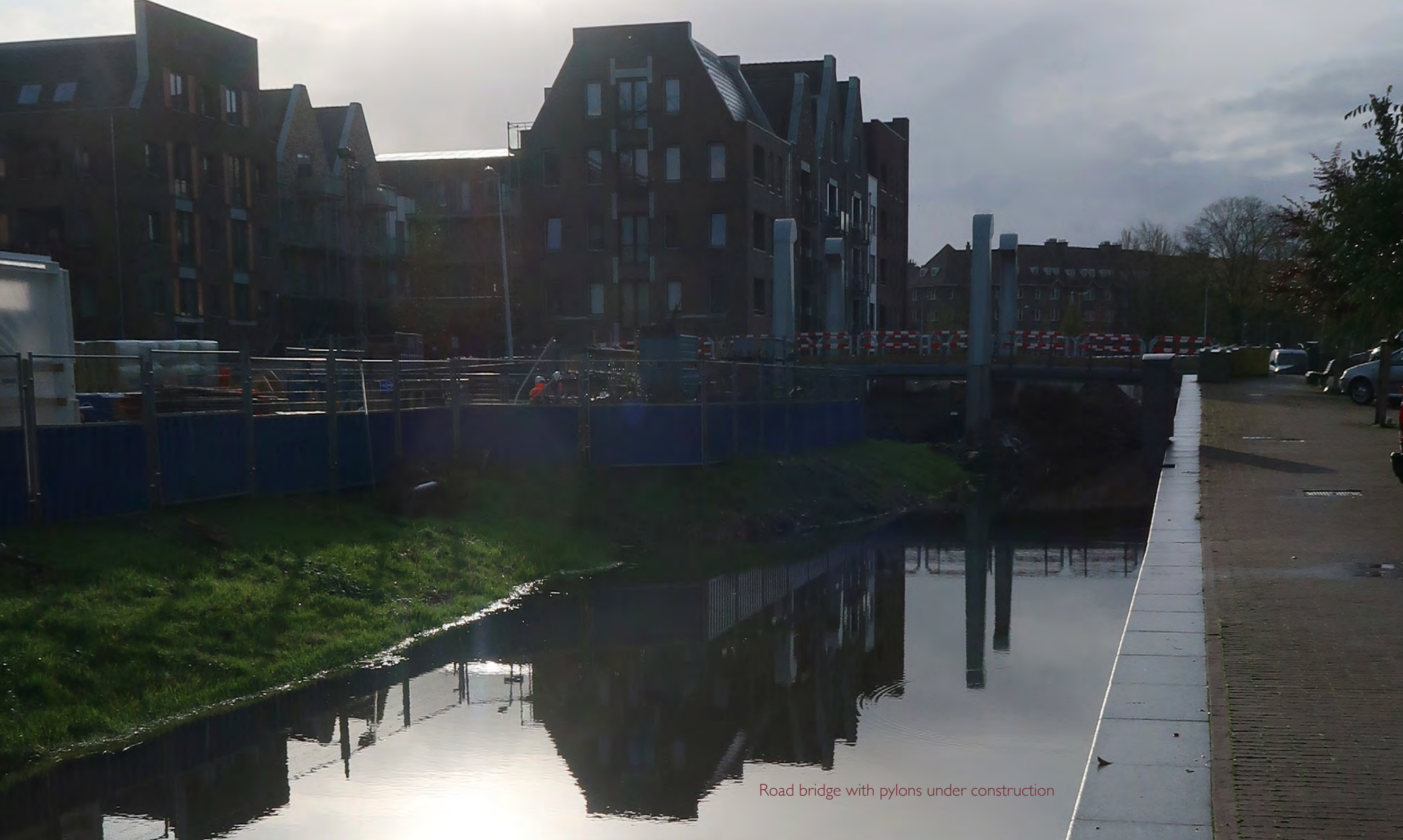
Bridge type A2: road bridge with a span of 20 metres, width 8.50 metres, clearance profile 2.50 x 5.00 metres
