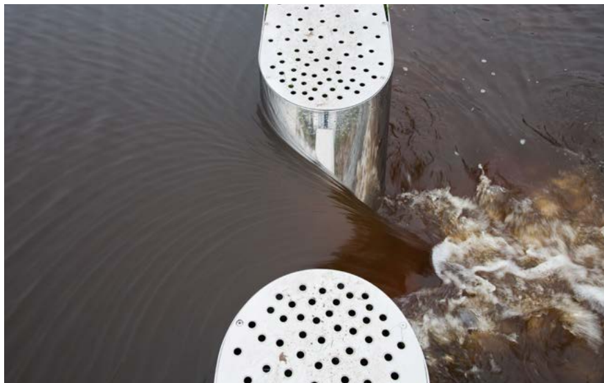
stainless steel step plates on the heads of the funnels provide a safe crossing
